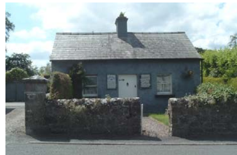
Vernacular random rubble wall, outside hairdressers
