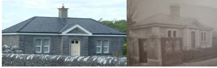
One of the two gate lodges, at the main entrance to Ardagh House today and in the nineteenth century. Note the difference in the way the uPVC windows (above) and the timber ones (below) open. Note how the cornerstones were once painted a light colour.
