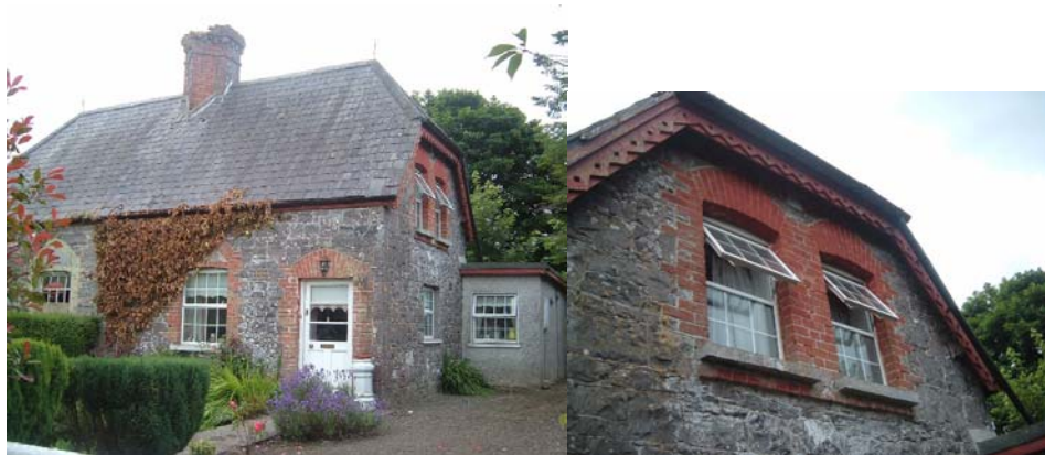
House 8, showing the kitchen extension and the new redbrick surrounds
