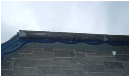
Timber soffit (Garda Station)
