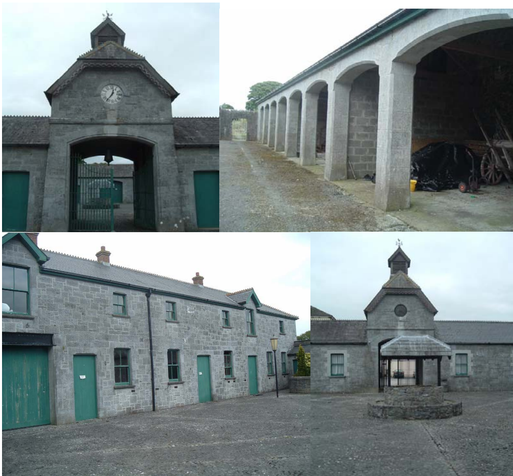
Various views of the stables. Note the half-hipped roof at the entrance, a style which is repeated in the Garda Station, and the semi-detached stone houses along the east road, and is copied in some modern houses. Note also the triangular arts-and-crafts-style dormers.
