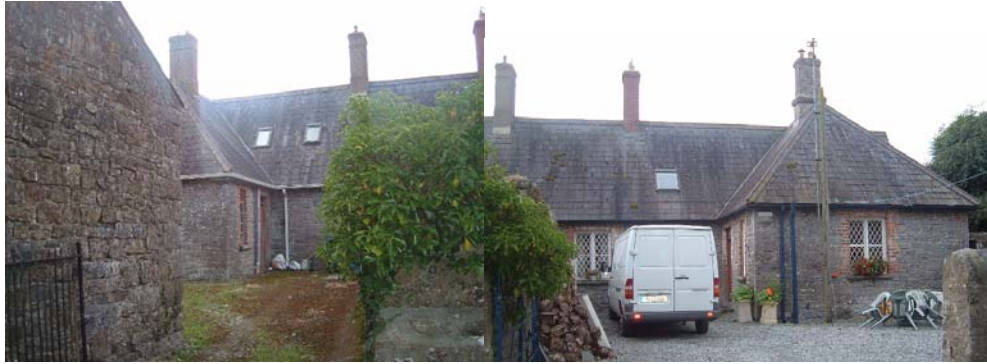
Behind houses 2 (left) and 3
