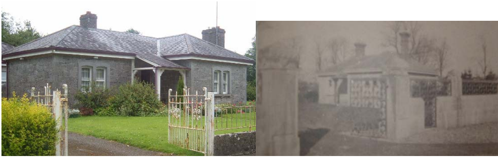
The other gate lodge, at the entrance on the east road. Note how the railings were once dark much darker than they are today.
