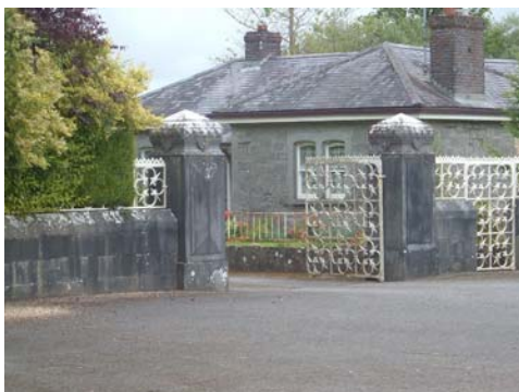
Gate to Ardagh House from east road
