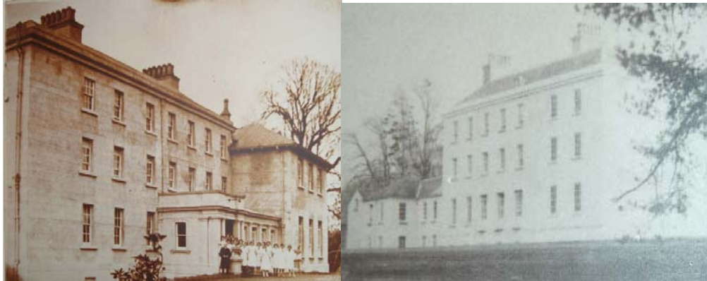
Ardagh House, as it was in the nineteenth century, front (left) and rear (right). Note how, in true Victorian style, the ashlar stone is visible. It is possible that the house was built this way, but it is also possible that the mortar was removed during the nineteenth century, because it was fashionable to show the stone, to make buildings look "old."
