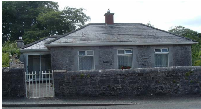
House 8: note the inappropriate entrance on the left
