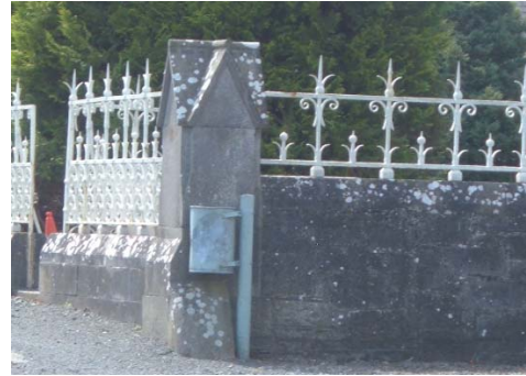
Pier around clock tower
