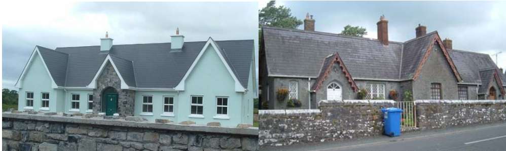
An example of recent development near Ardagh village. Note the architectural paradigms similar to those in the old buildings nearby (triangular gables, use of symmetry, use of stone, pitch of roof etc).
