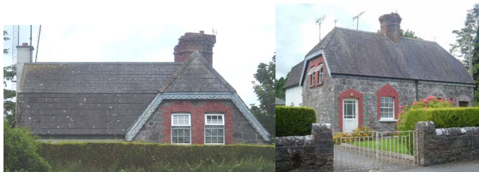
The extension to the rear of house 5 (on the left, perpendicular to the original house)
