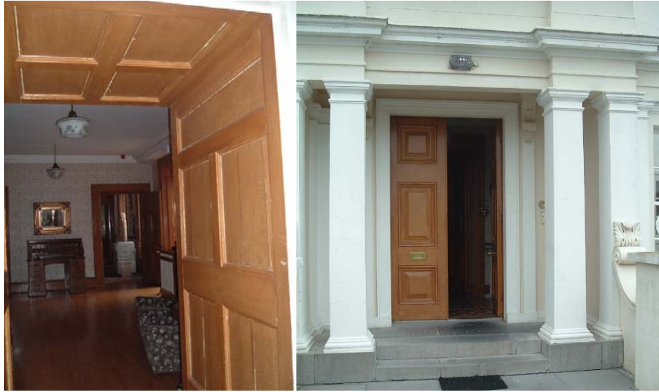
Wooden panelling in a doorway and the Doric columns in the grand entrance.
