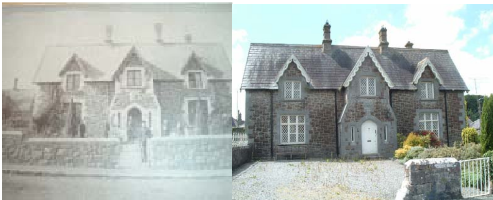
Once the RIC Police Barracks, now a rented house (although currently uninhabited). The photos suggest that little has changed, and this is probably the best example of how the houses once looked.
