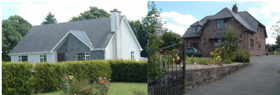
Houses 8 (left) & 10. Note the half-hipped roof, which resembles that of the Garda Station building
