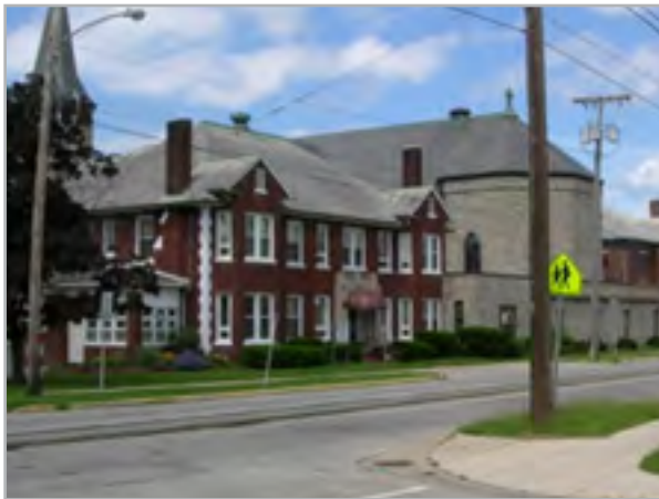
St. Mary's Church and Rectory, 411 W. 11th Street
