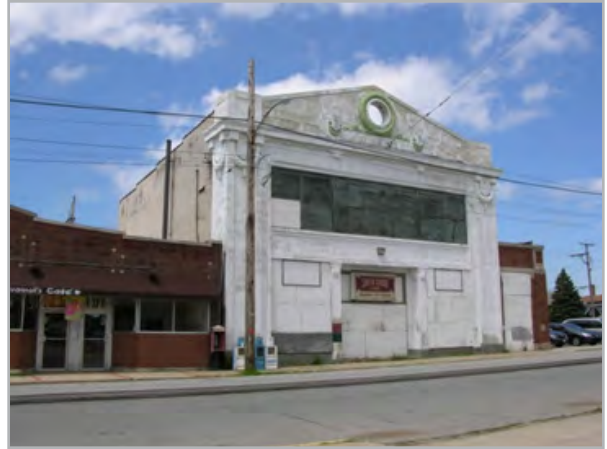
South Shore Station, 11th Street
