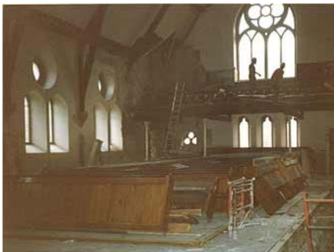
The original pews also had to be cleared.
