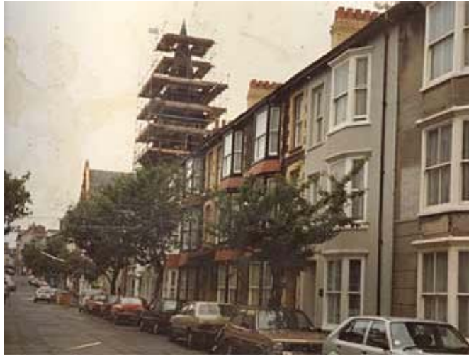
← Scaffolding was erected around the original spire. →
