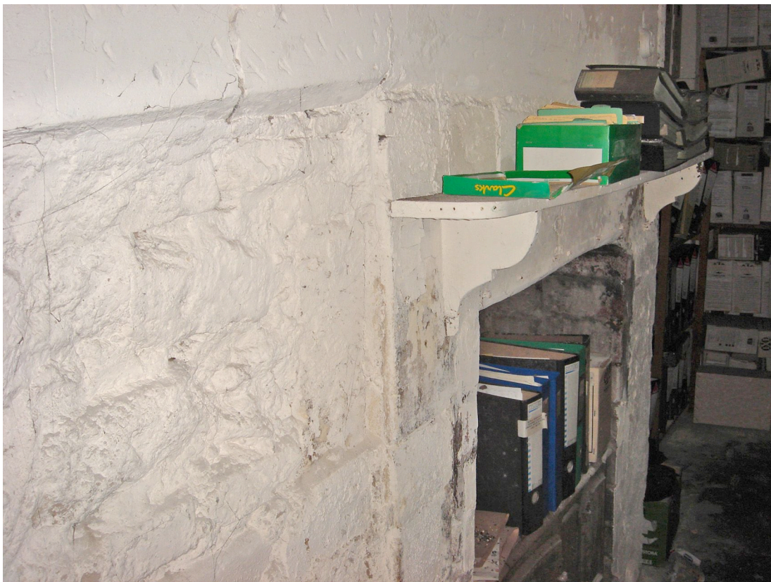
The blocked-in Tudor fireplace in the cellar of the Ralph Allen Town House, with a smaller fireplace inserted into the right side. See also page 54.
