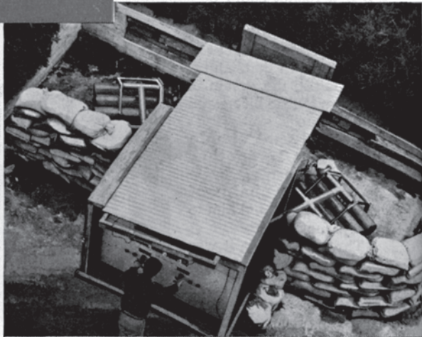
To determine stability, a flying model is fired with powder by remote control, top. Center, recoil of spring gauges strength of powder fuels. Behind the sandbags (bottom) California Institute of Technology scientists test rocket motors and explosive fuel—mixture of oxygen and ethylene—developing 5,000-degree heat and gas velocities of 3,600 miles per hour
