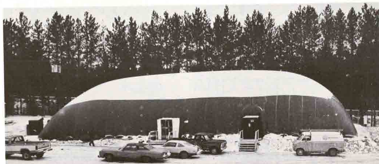
Modern air inflated buildings were used as press subcenters at Mt. Van Hoevenberg and Intervale ski jump complex
