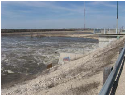
Figure 8-C: The Red River Floodway Gates
