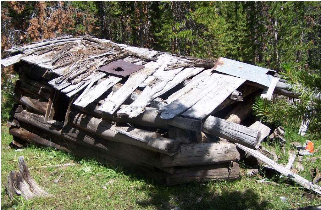
Photo # 1 (Utah_Summit County_Archie Creek Camp_0001.tiff): Feature 1: South elevation, camera facing northeast.
