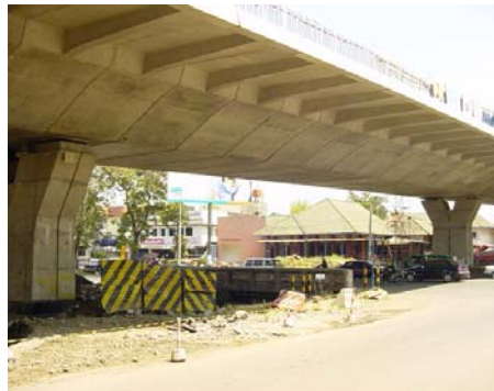
▼ Underneath view of viaduct
