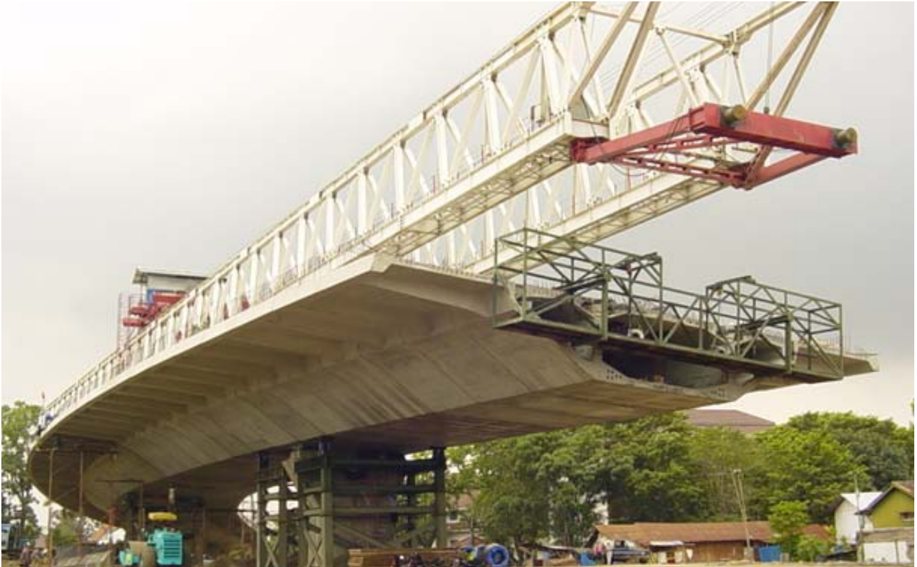
▲ Curved section of east viaduct
