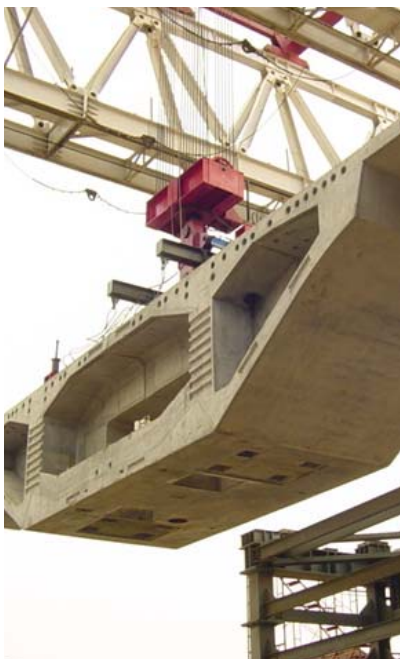
▼ Pier segment erection
