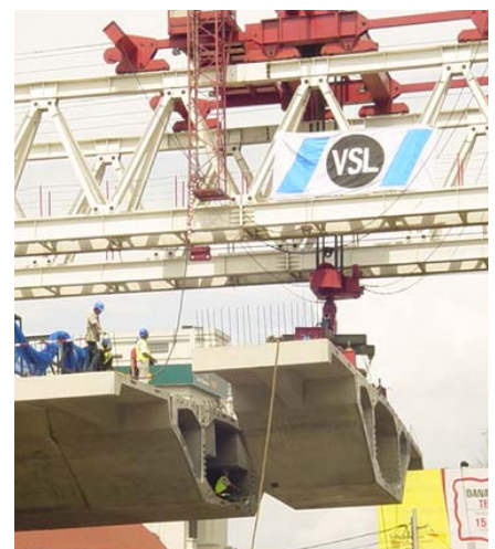
▲ Field segment erection at Jl. Dago
