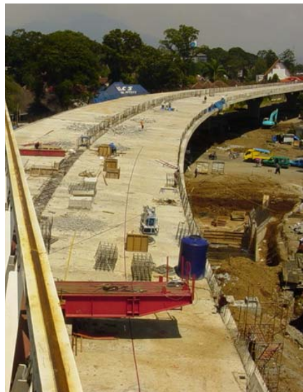
▲ Top deck view of east viaduct
