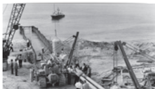
Construction of Arish Mell pipeline begins
