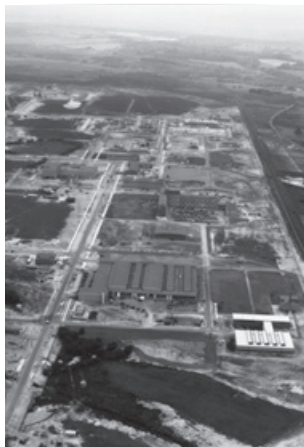
Work on the Winfrith site begins
