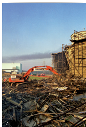
4 SGHWR cooling towers demolition 1991
