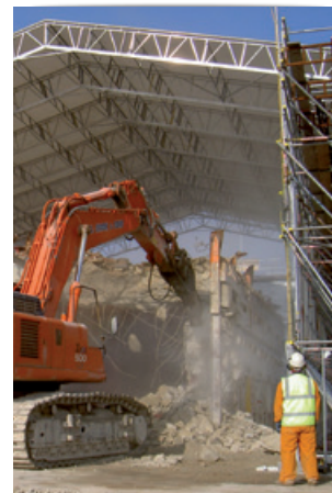
Active handling building demolished
