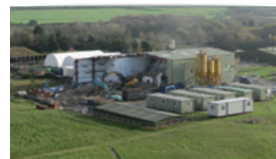
Demolition of WETP
