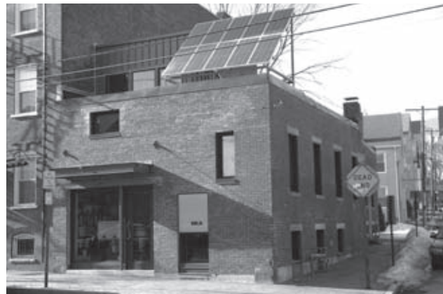
This contemporary design by architect Richard Renner integrates solar panels into the rehabilitation of a former commercial building in Portland.
