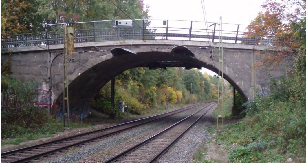
Figure 1.1: The Glomman Bridge.
