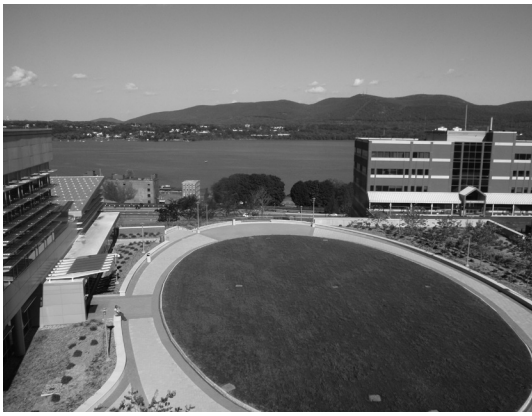
Green roof at SUNY Orange in Newburgh
