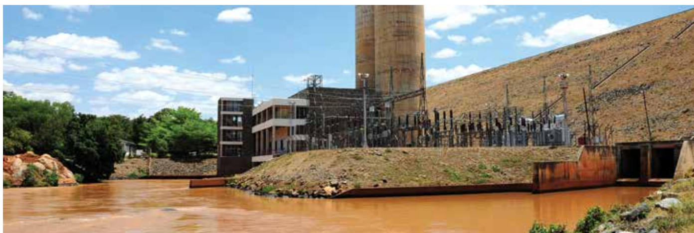
Masinga Power Station in the 7 Forks Cascade. It holds approximately 2 billion litres of water making it KenGen's largest dam in the Eastern Hydros area
