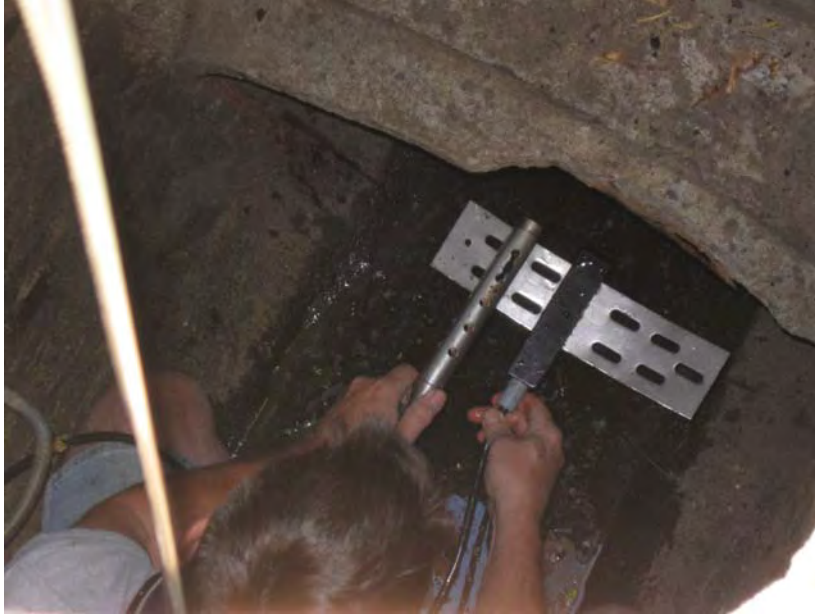
Figure 25-3. The AV probe and intake strainer being anchored to the invert.
