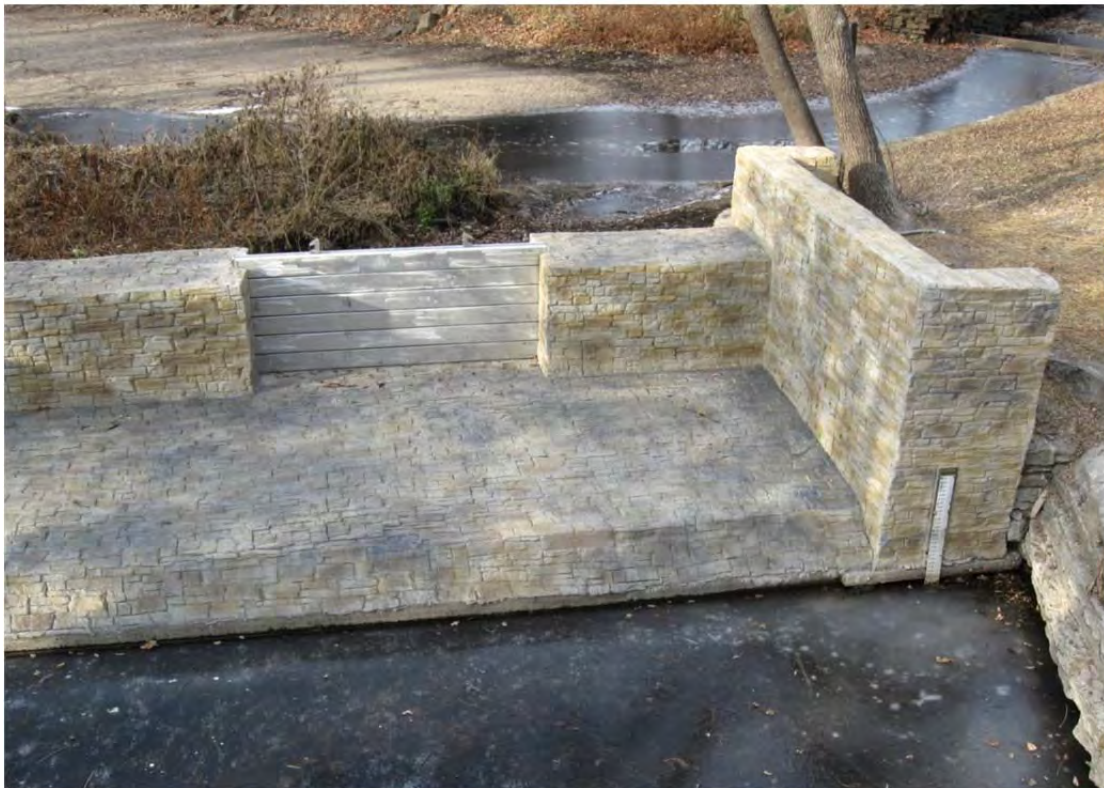
Figure 12-1. Newly constructed weir at Lake Nokomis outlet, taken November, 2012.
