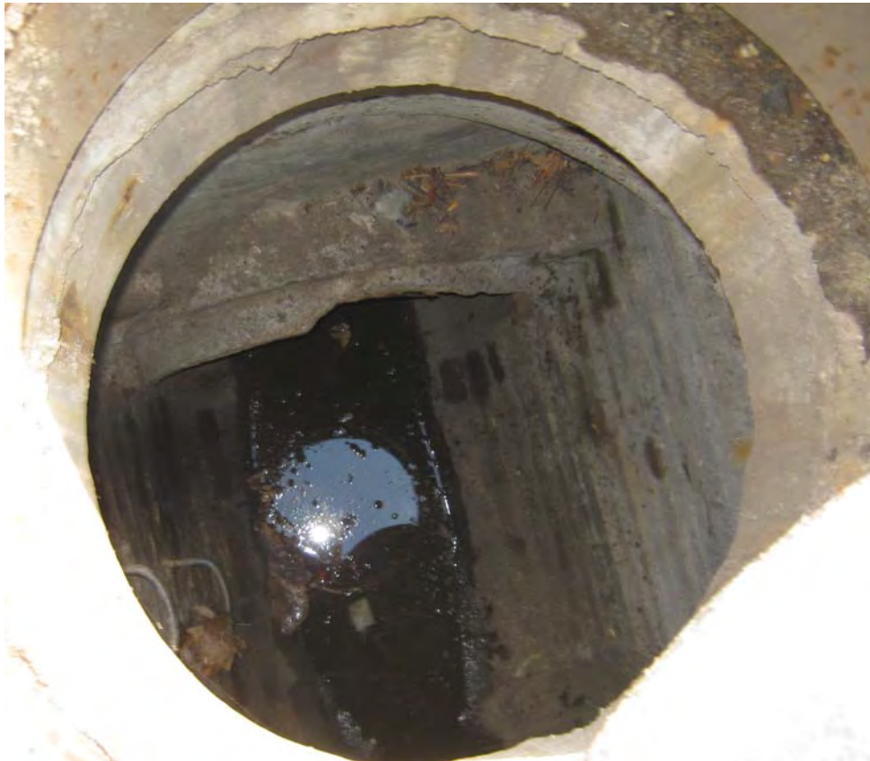
Figure 25-2. The manhole street view of the 56 th and 21 st 30” pipe.
