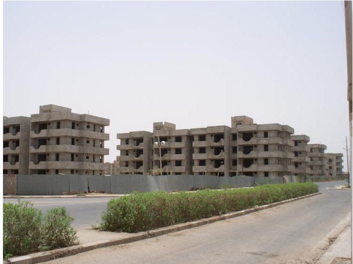
Figure 19. Construction in residential buildings, mainland-Massawa, 2011
