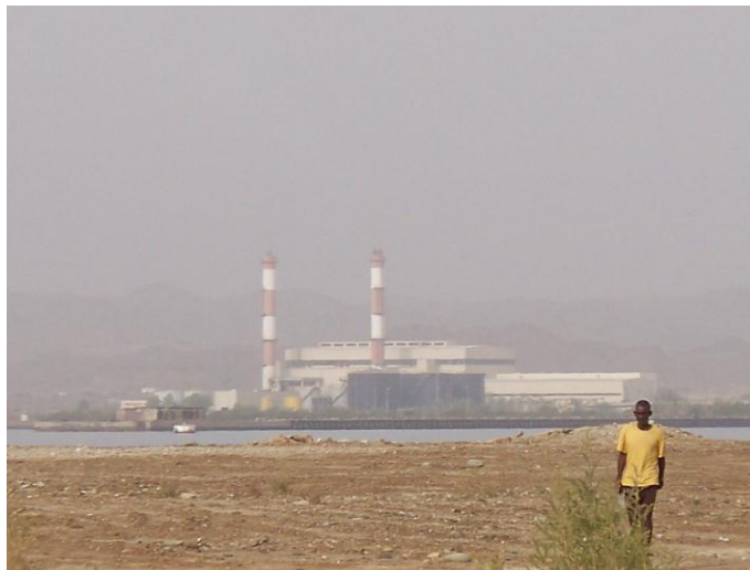
Figure 20. Hirgigo power plant from Tualud island, Massawa 2011
