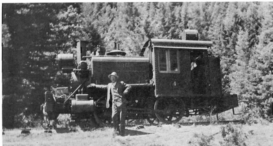
Albion Lumber Company engine Number 4 at Wendling in July, 1937, while being used to tear-up the Albion Branch.
