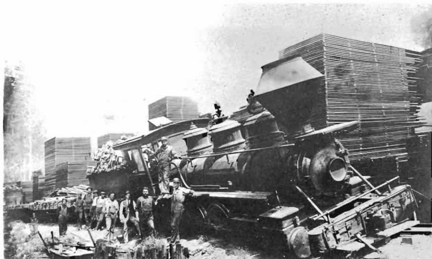
Northwestern Pacific Railroad engine Number 226, 0-6-0, derailed while switching the lumber yard at Navarro.
