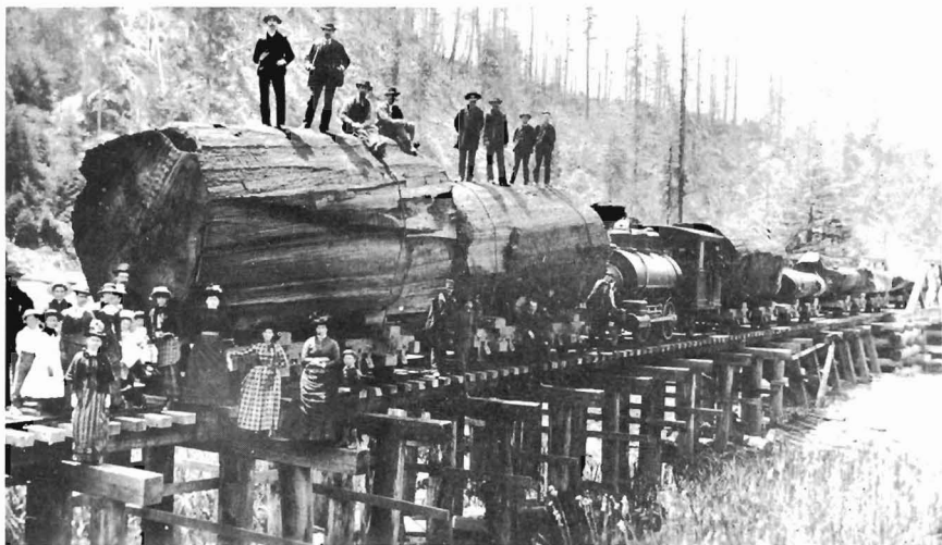
Albion River Railroad train with engine Number 1, 2-4-2T, sandwiched in the middle in 1892. Collection of B. H. Ward
