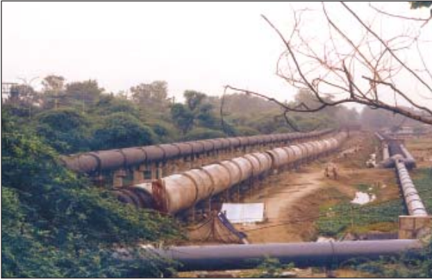
Pipeline from Muradnagar to Sonia Vihar
