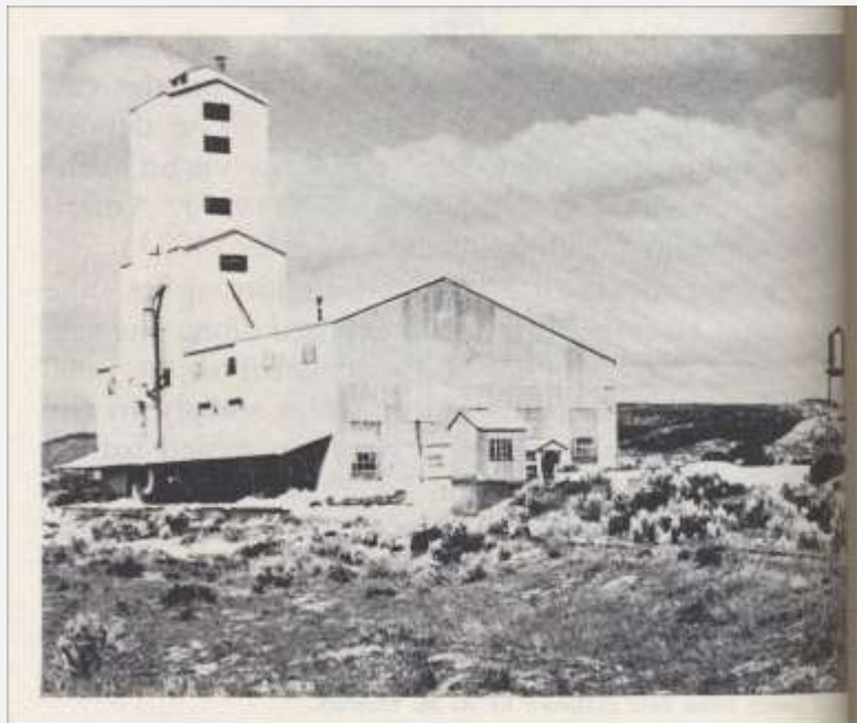
“Photo 32.... Pacific mill, just east of Cameron Corners and adjacent to San Diego and Arizona Eastern Railroad. Feldspar and quartz from the Pacific mine, about 5 miles to the northwest, were milled here until 1943. The Campo Milling Corporation operated the mill in the early 1950’s.) (pp. 76)
