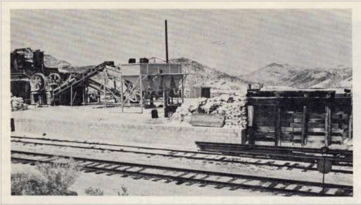
“Photo 49. View north across limestone milling equipment at Dos Cabezas siding toward Heathman crystalline limestone deposits in low hills in background. Principal quarry (photo 50) is visible just to left top of wooden loading ramp.” (pp. 178)
