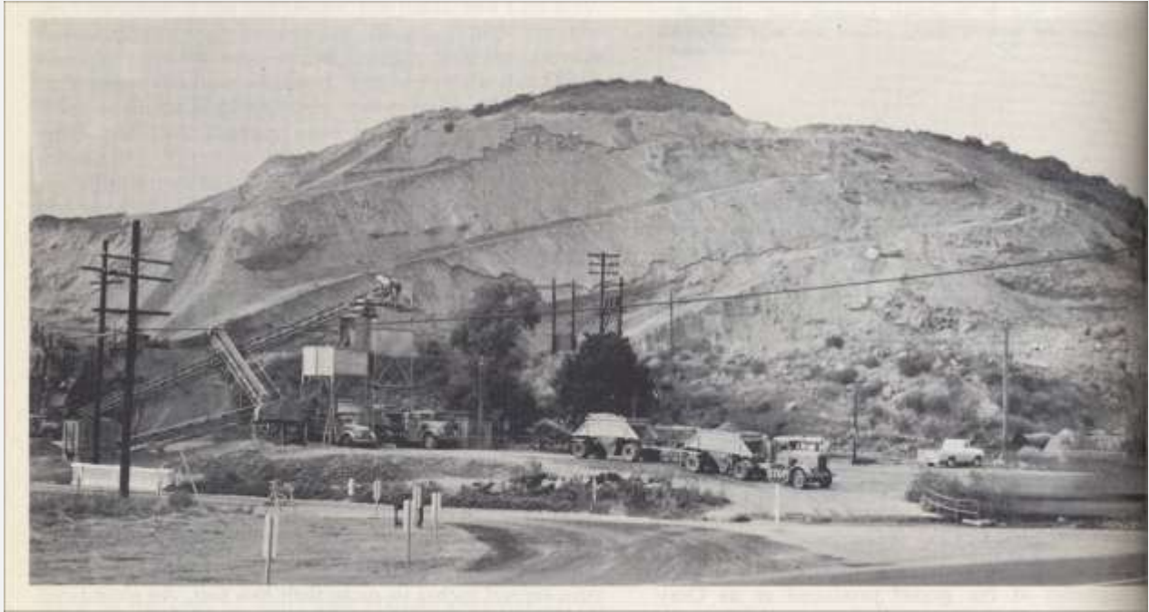
“Photo 74. Decomposed granite operation at Jamacha Junction of San Diego Cement Company subsidiary of Caudell and Johnson; view southwest. Tractor scrapers shave ‘DG’ into bunker (left); oversized boulders are discarded in area shown at right edge of photograph. From bunker, material is either transported by belt to mill shown above, or used without processing.” (pp. 230)
