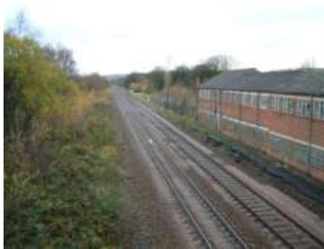
Looking Towards Dronfield from Unstone Station Site.
