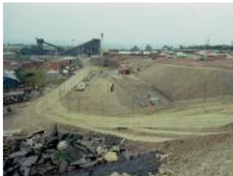
Construction of the No. 3 Drift. (Brian Crossland). A modern drift mine.
