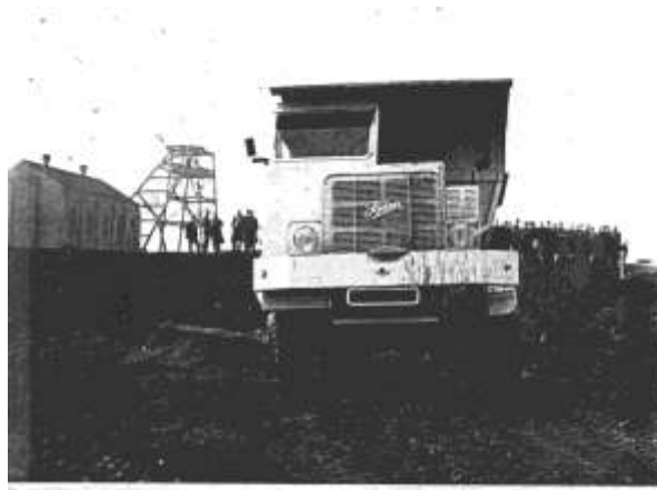
New Dumpers. New Shaft.
