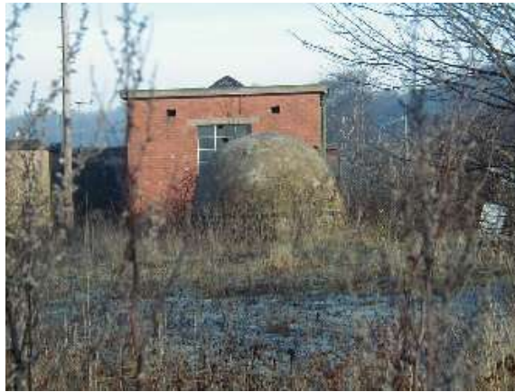
Capped off Shaft on the Works. (ANB).
