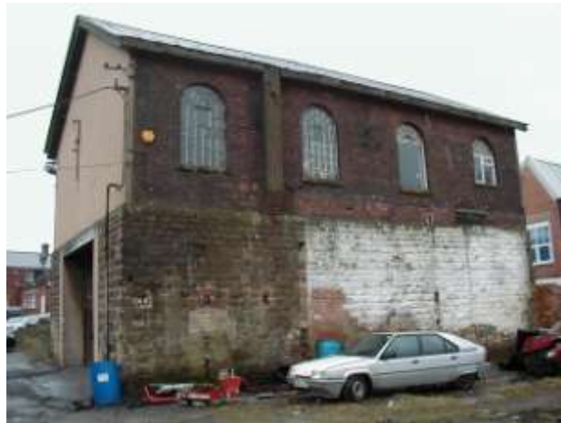
Sheepbridge Colliery (Possibly) Winding House.
