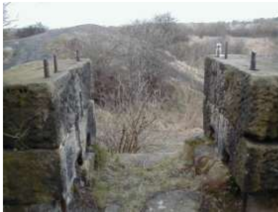
Remains of No. 11. Avenue. (Possibly to do with Winding). (ANB).
