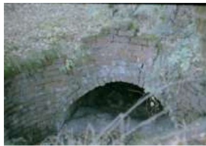
Upcast Shaft and Entry to Ventilation Drift. (ANB).
