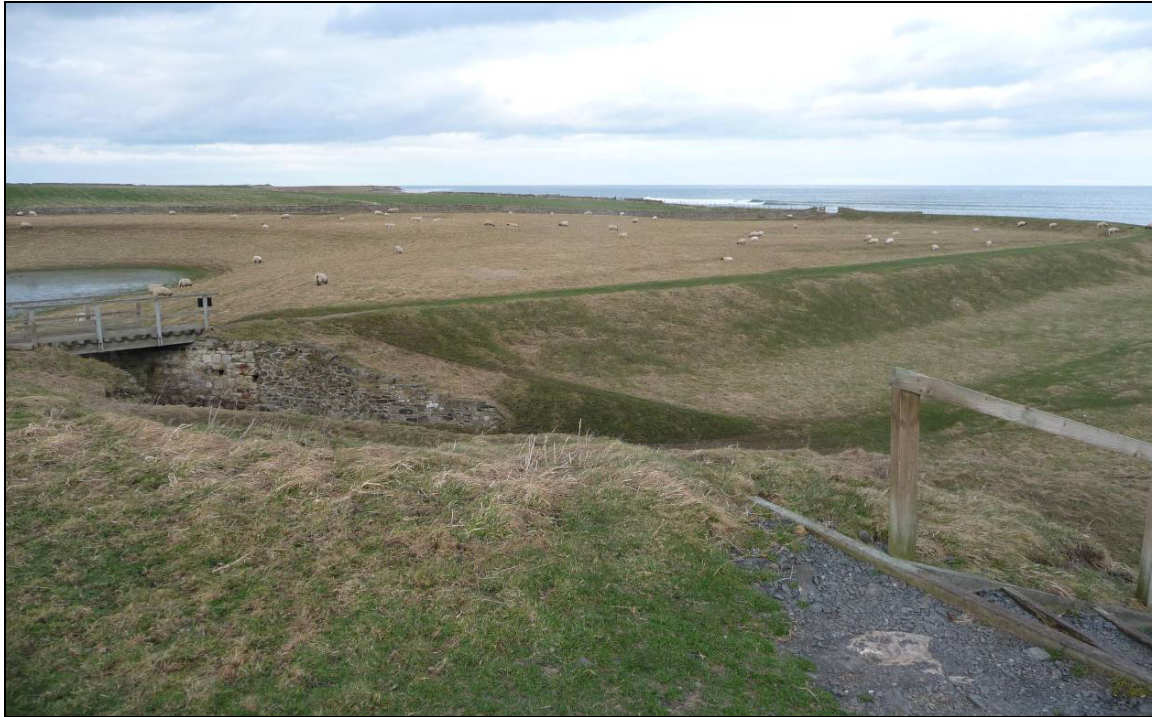
Plate 14. Waggonways built to carry limestone from the quarries to the kilns
