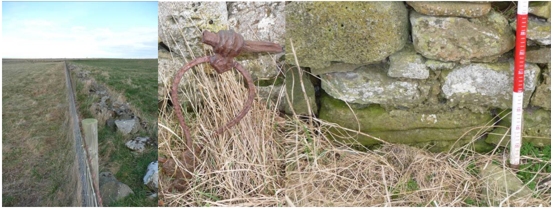
Plate 10. (i) The replacement of walls with post and wire fencing will lead to a change in historic character. (ii) Iron bedsteads provide an ornate solution to stockproofing. (iii) a rock in the wall shows signs of having been upright with rainwater eroding down its face before being used to build a wall in the 18 th century.
