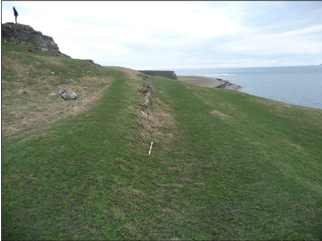
Plate 12. Access tracks to the top of the limekilns
