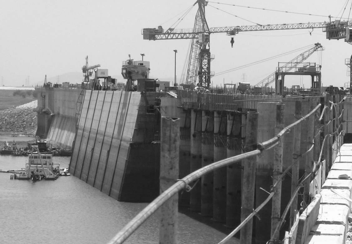
Raising the height of the Roseires Dam on the Blue Nile, April 2009 Courtesy Donielle DeToy and Hussein Askary
