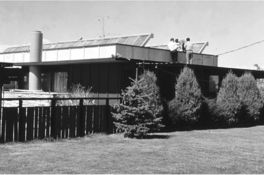
Fig. 16: The Denver house, designed by Hunter and occupied by the Löf family since 1957
