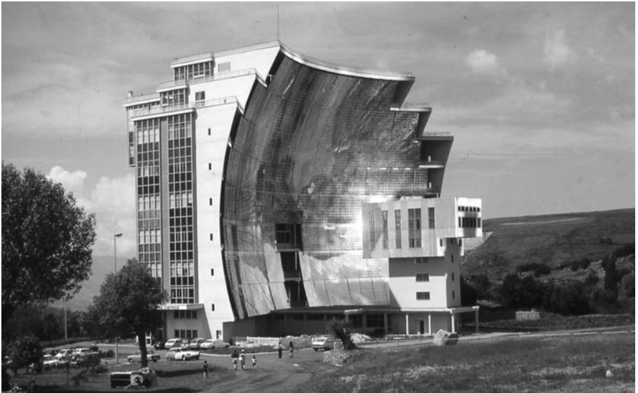
Fig. 10: The Montlouis 50m solar furnace. The proposed AFASE furnace was to be of similar but smaller design
