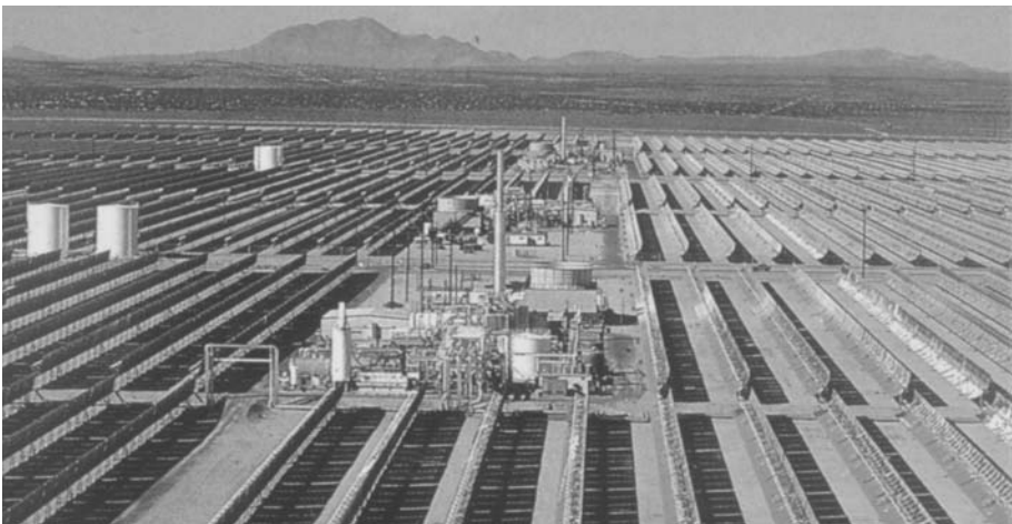
Fig. 4: One of the LUZ solar thermal power plants in California
