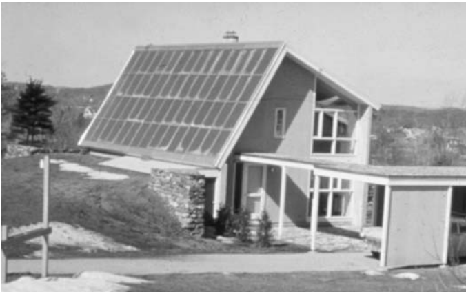
Fig. 17: MIT House IV, with liquid heating collectors and water storage
