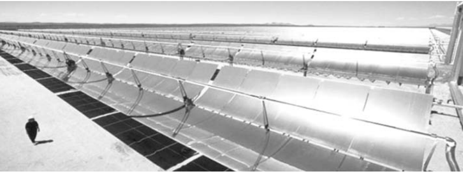
Fig. 3: Detailed view of the LUZ collectors in a California solar thermal power plant. There are more than a million square meters of collectors in the several plants. The receivers utilize selective surfaces and are enclosed in vacuum jackets.
