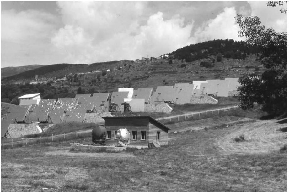
Fig. 11: The heliostats for the Montlouis furnace (not aligned when photo was taken)
