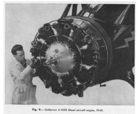
A later Guiberson. Diesel is the A-1020 model which is similar to its predecessors but has up-to-date valving (Fig. 9). This engine passed its civil government tests in 1940 and was awarded A.T.C. No. 220 with a rating of 310 h.p. at 2,150 r.p.m. It weighs 650 lb., or 2.1 lb. per h.p.
