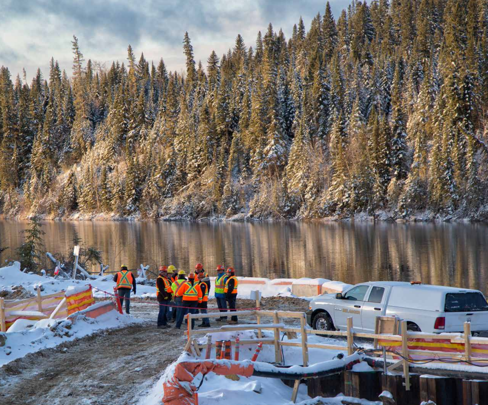
Peter Sutherland Sr. GS worksite
