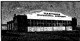
Hastings Municipal Airport Hanger at West 12 th Street (AD04-003)
