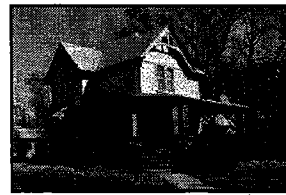
House at 701 East 2 nd Street (AD04-491)
