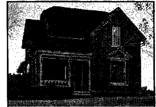
Queen Anne style residence, Juniata (AD08-006) – potentially eligible for the NRHP
