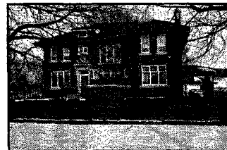
House at 1136 North St. Joseph Avenue (AD04-265)
