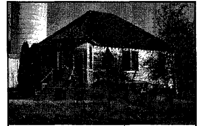
Lincoln Avenue and 2 nd Street, Ayr (AD02-004) – potentially eligible for the NRHP
