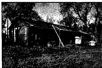
Jackson-Einspahr sod house (AD00-057) – potentially eligible for the NRHP
