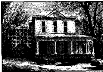
House at 722 North Hastings Avenue (AD04-231)
