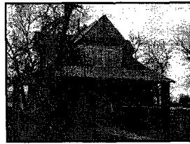
Thomas Trausch Residence on the south side of Davis Street (AD12-004)
