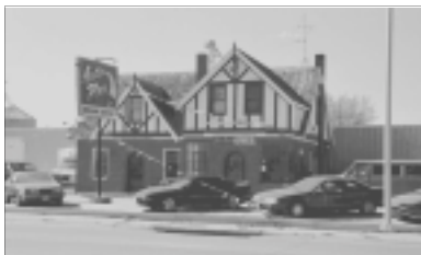
Commercial Building at southwest corner of Sheridan and Lincoln Streets, West Point (CM05-157)
