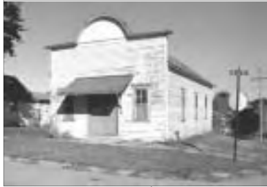
Commercial Building, 4 th and Main Streets, Beemer (CM03-003)
