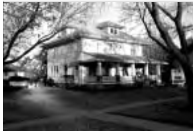
House at 143 South Farragut Street (CM05-126)
