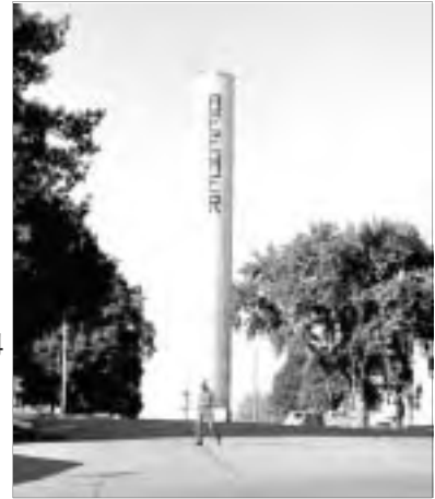
Water Stand Pipe, Beemer (CM03-032)
