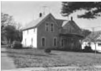
House at 705 Main Street (CM02-012)
