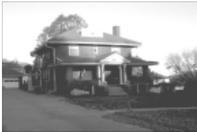
House at 207 South Farragut Street (CM05-125)
