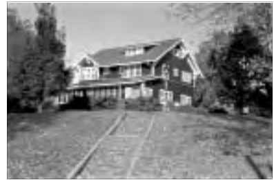
House at 230 South Farragut Street (CM05-124)
