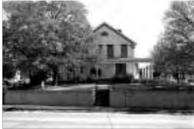
House at 606 North Lincoln Street (CM05-022)
