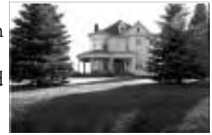
House at 302 Grove Street, Bancroft (CM02-003)
