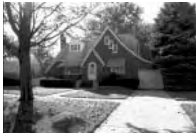
House at 417 South Monitor Street (CM05-116)
