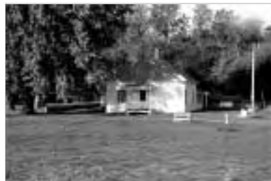
One-story Cube House Located on Farmstead, Bancroft (CM00-191)
