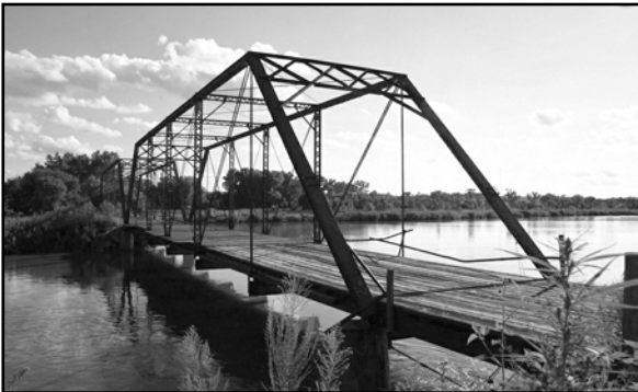
Sargent Bridge near Sargent, CU00-073, listed in the National Register
