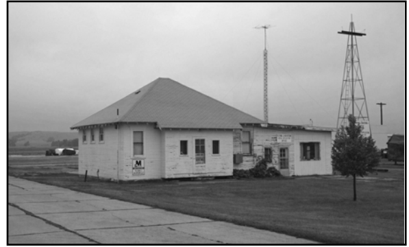
Broken Bow Municipal Airport near Broken Bow, CU00-092
