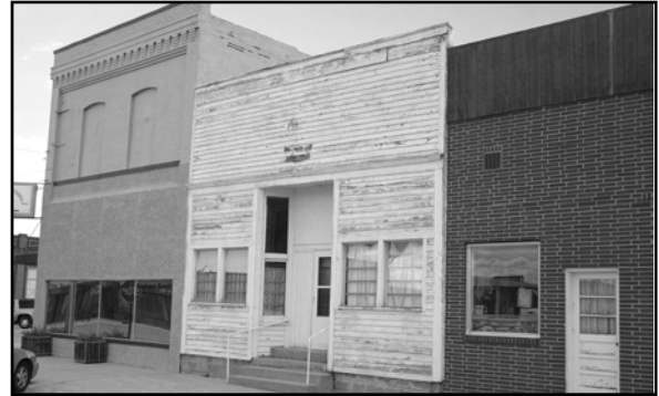
Commercial building in Arnold, CU03-020
