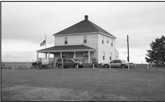
American Foursquare house near Callaway, CU00-025
