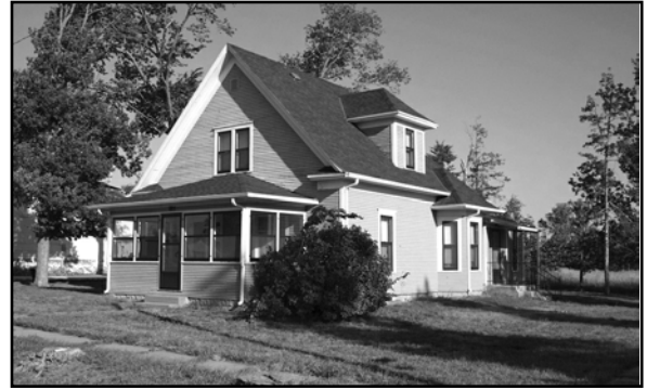
Front gable house in Oconto, CU14-021
