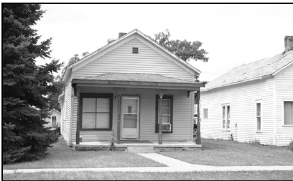
Front gable house in Callaway, CU06-031
