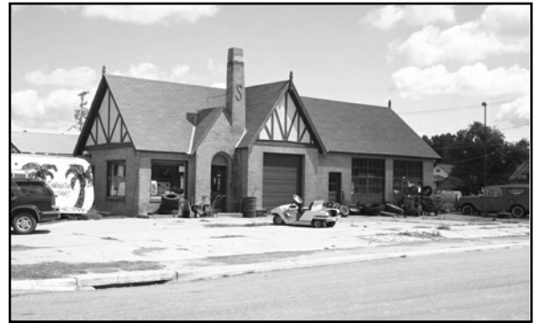
Service station in Sargent, CU17-036
