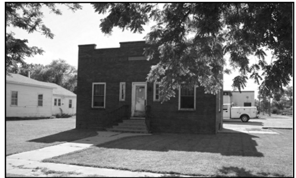
Telephone Office in Sargent, CU17-046 Diversion
