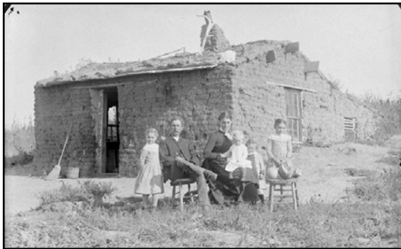
Sod house with a sod roof (NSHS)
