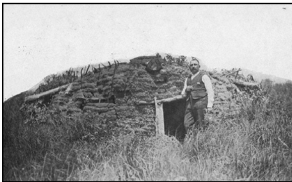
Example of a dugout constructed of sod (NSHS)
