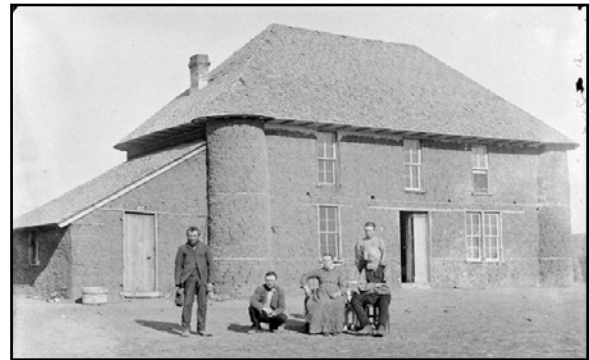
Two-story sod house (nonextant) built by Isadore Haumont in Custer County (NSHS)
