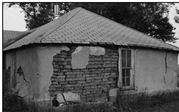
Sod house with stucco exterior identified during field survey, CU00-021
