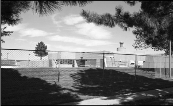
Melham Park Pool Building in Broken Bow, CU05-160
