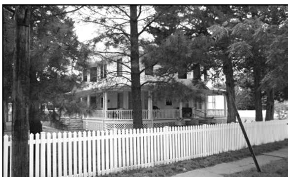
Vernacular house in Callaway, CU06-013
