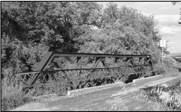
Victoria Creek Bridge near Anselmo, CU00-075
