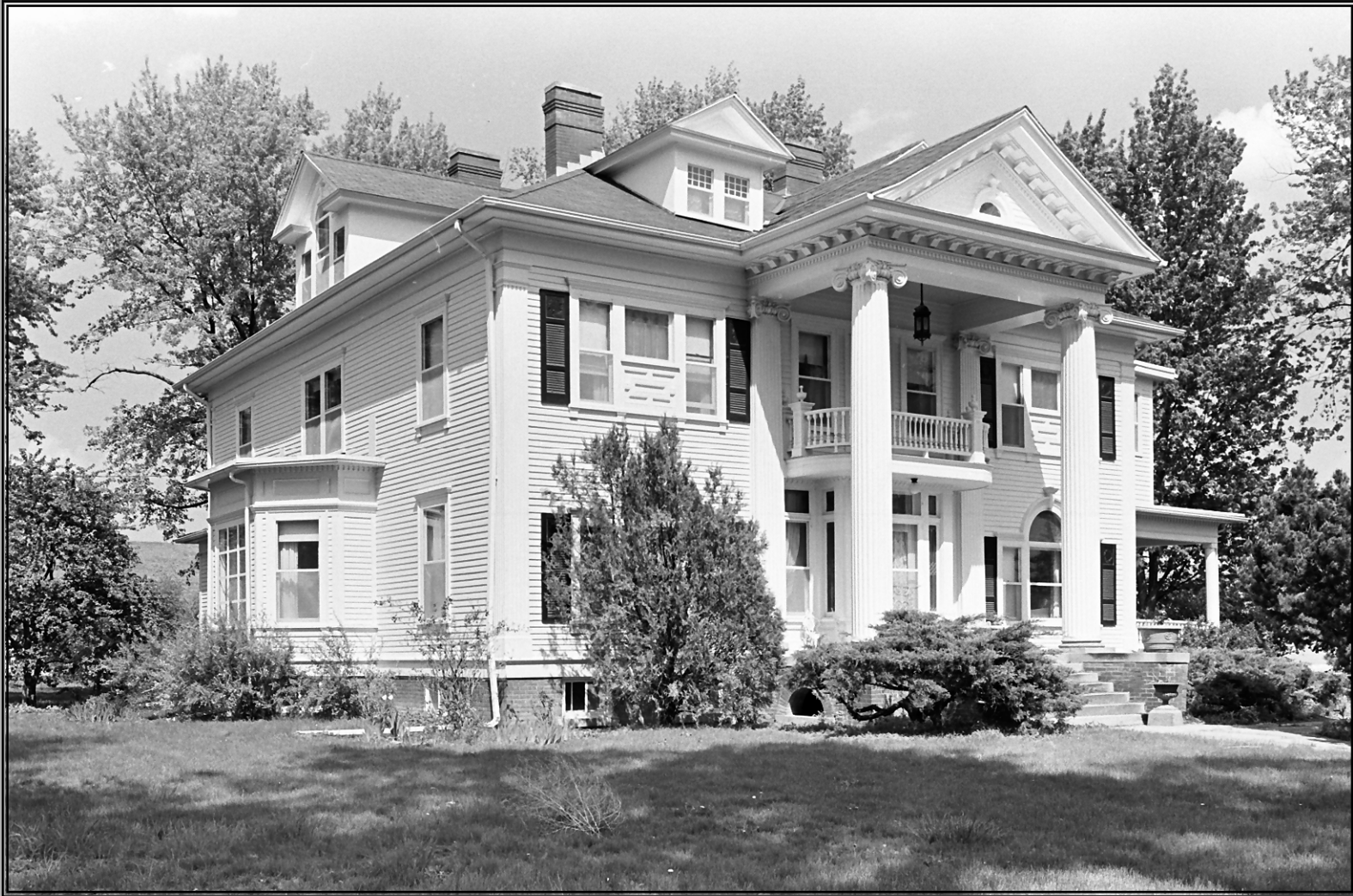
Photo 1 of 8—general view looking east.
