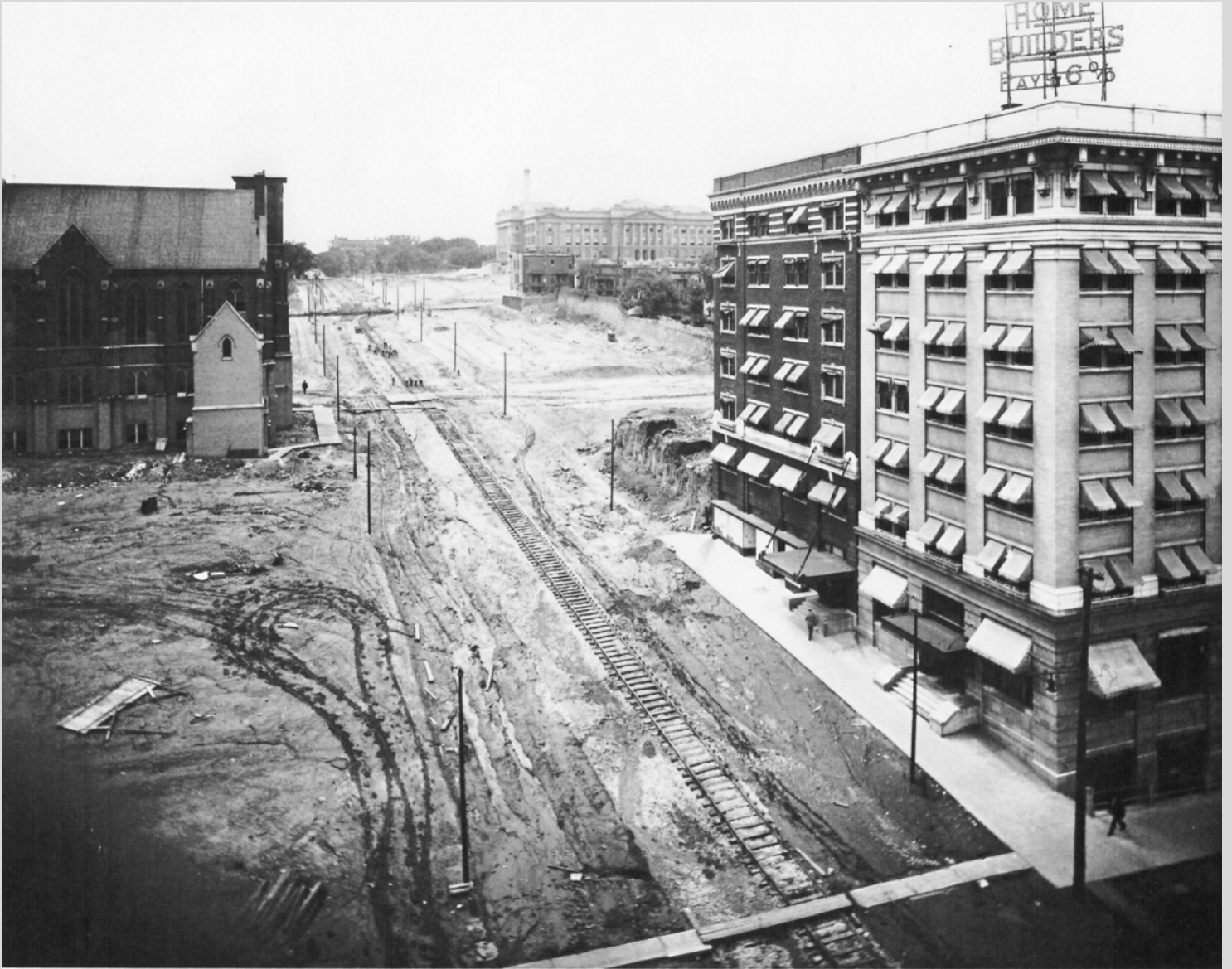
The Logan during street construction.
