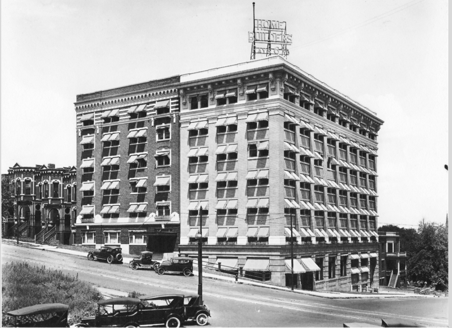
The Logan before street construction.
