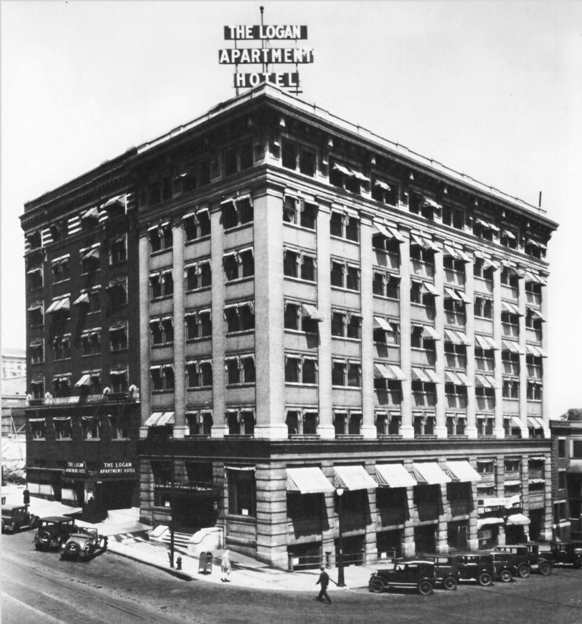
The Logan after street construction
