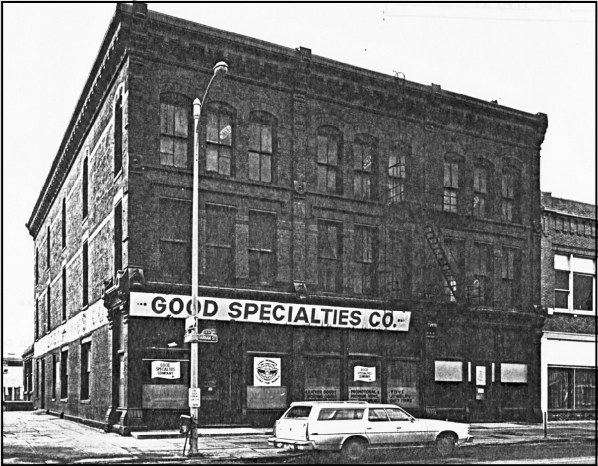
Photo 1 of 2 — view of north façade, looking southwest. Photo by Lynn Meyer, 1977, Landmarks Heritage Preservation Commission, Omaha
