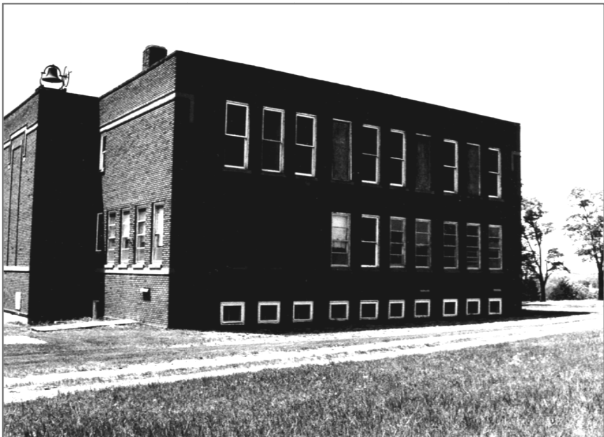
View looking NW Photo by Carol Ahlgren, June 1997, NSHS (9706/1:22)
