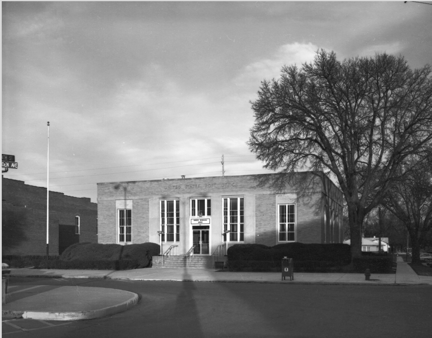
Photo 1 of 3 — view looking northwest showing south and east facades Photo by Jeffrey Bebee, Oct. 1989, NSHS (H673.5-4914)
