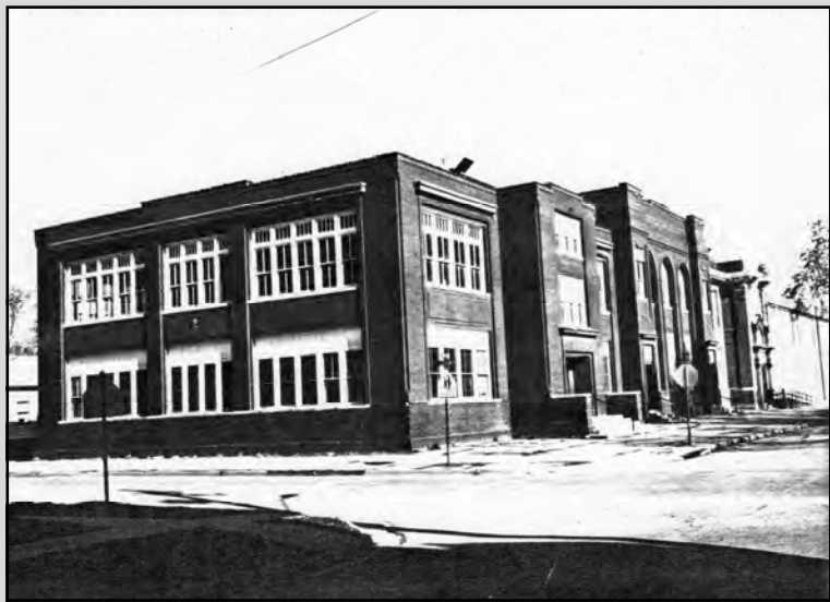
Photo 1. South and east facades looking northwest (8504/3:35)
