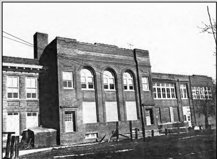
Photo 6. South portion of west façade, built 1923, looking south-east (8504/3:26)
