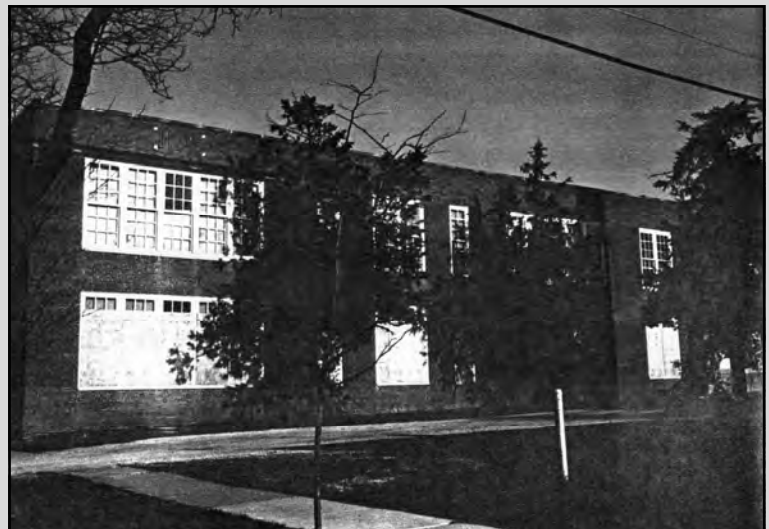
Photo 4. North portion of west façade, built 1925-6, looking south-east (8504/3:22)
