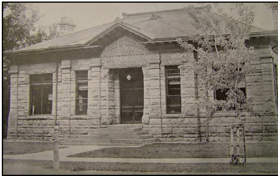
Figure 11. Andrew Carnegie provided $10,000 for the construction of the 1902 sandstone library on Macon Avenue designed by Charles C. Rittenhouse. SOURCE: Cañon City Chamber of Commerce, Cañon City, Colorado (c.1920s).
