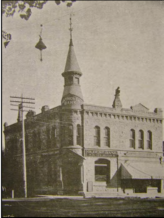
Figure 7. The Raynolds-McGee Block (1883) housed the Fremont County Bank until 1921 and was built of Castle Rock rhyolite and stone from areas near Canon City. SOURCE: Picturesque Canon (1892).
