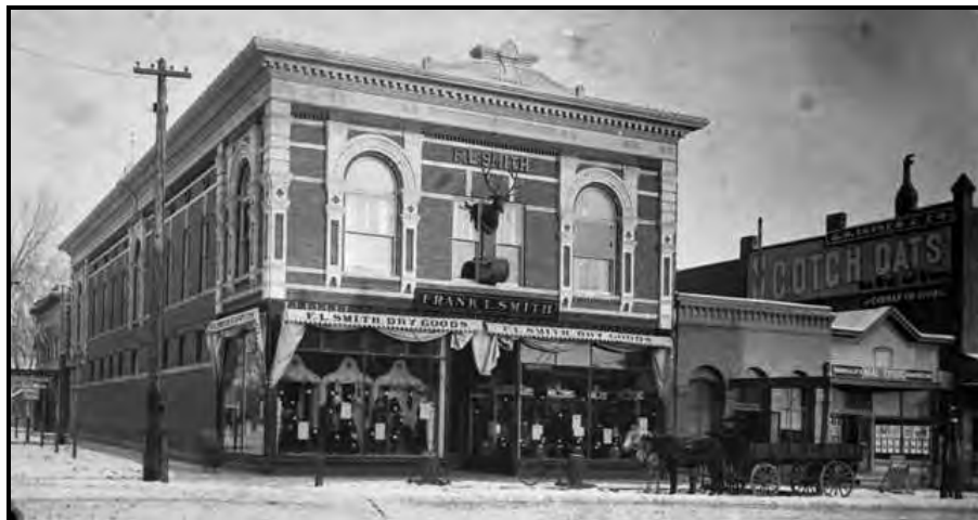
Figure 10. Architect Charles C. Rittenhouse designed this building for Frank L. Smith's dry goods business in 1901. Initially the Elks leased the upstairs hall. In 1927-28, the Knights of the Ku Klux Klan held its meetings there. SOURCE: Denver Public Library, Western History and Genealogy Department, Image Number X-6995.
