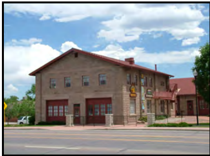
Former fire station, Royal Gorge Blvd.
