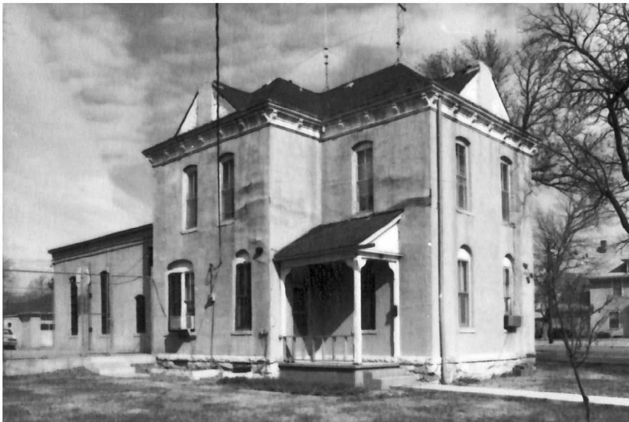
Photo 3 of 3 — Jail, looking northwest showing east & south facades Photo by BJB Long, Four Mile Research, 1989 (NSHS 8904/9:30)
