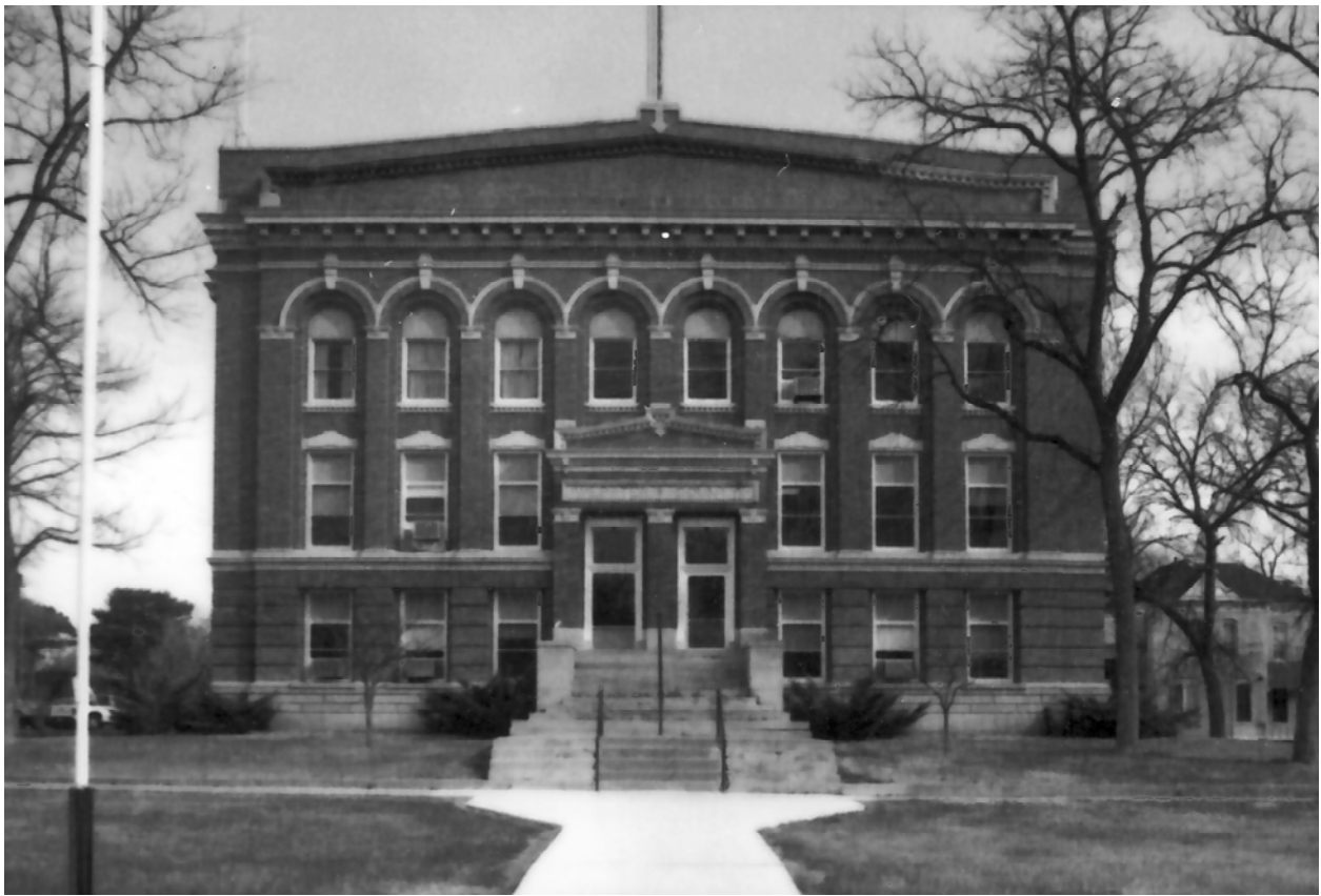
Photo 1 of 3 — view looking north showing south façade of courthouse, jail to right Photo by BJB Long, Four Mile Research, 1989 (NSHS 8904/9:20)
