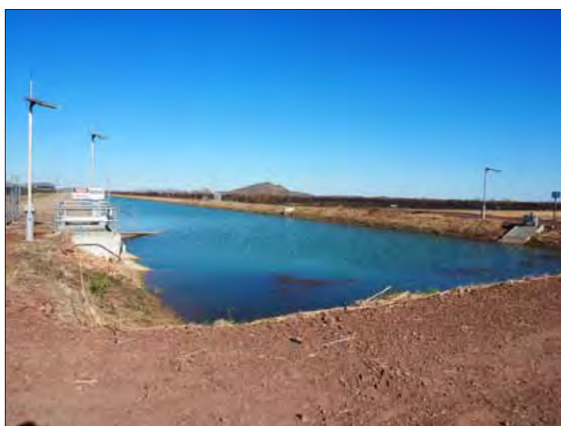
THE END OF THE LINE: The Commonwealth and Western Australian Governments have invested more than $500 million to bring the Ord Stage 2 irrigation channels within six kilometres of the Northern Territory border.
