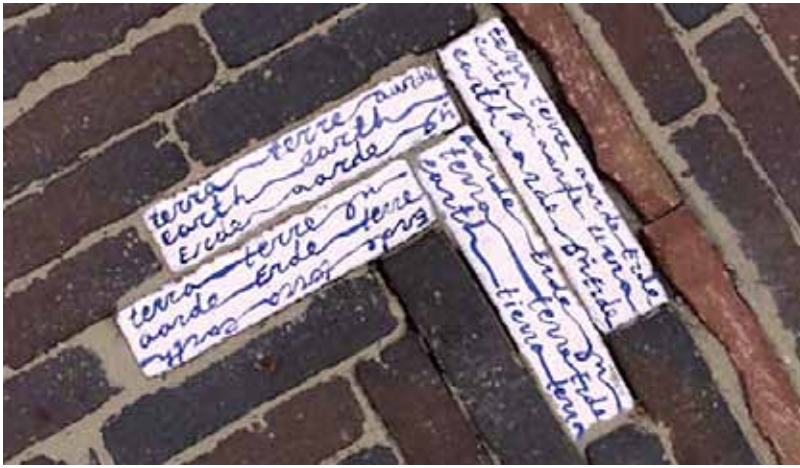
2011 Installation of the Ceramics Route: the glazed paving bricks in the historic center of Delft form a route leading past ceramic highlights. Each brick was decorated by hand by Christina Linaris Coridou and features the word 'earth' in different languages.
