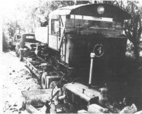
Close to fifteen years later, construction machines and a truck yank No. 4 from storage at Caguas. DAVID D. DEYO
