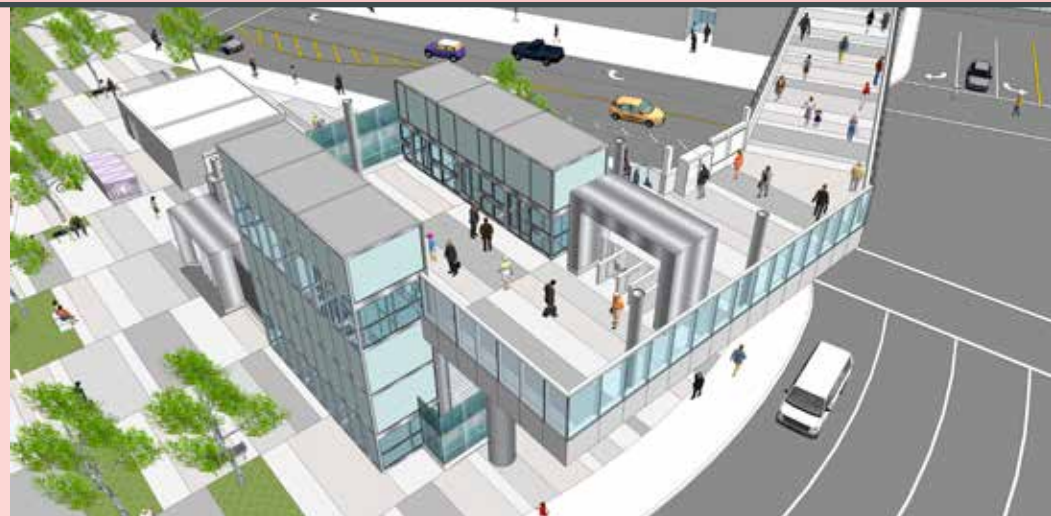
The 2nd/Hope Station Pedestrian Bridge Option would take pedestrians up one story, approximately 22 feet above Hope St. The bridge would connect to a new plaza currently under construction above General Thaddeus Kosciuszko Way (GTK Way) furthering the connection to Upper Grand.
