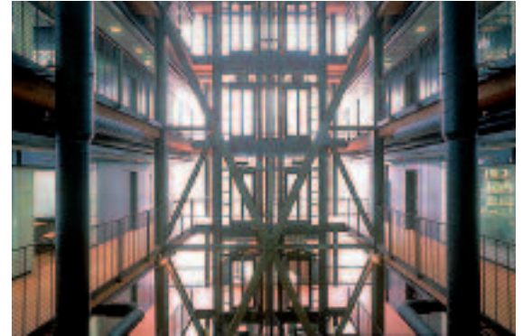
Abb. 6: Ungeschütztes Stahltragwerk, Administrative Office Building Arcelor Long Commercial, Differdingen, Luxemburg
