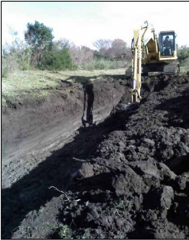
FIGURE 3. Heavy machinery opens a secondary course of the Vizcaíno stream to divert water away from the bone bed for the 2011 excavation. Photograph by Jean Philippe Gibert.
