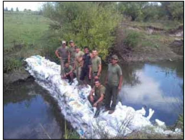
FIGURE 4. Members of the 14th Battalion of the Uruguayan Army pose on top of the dam they built for the 2011 excavation. Photograph by Richard A. Fariña.
