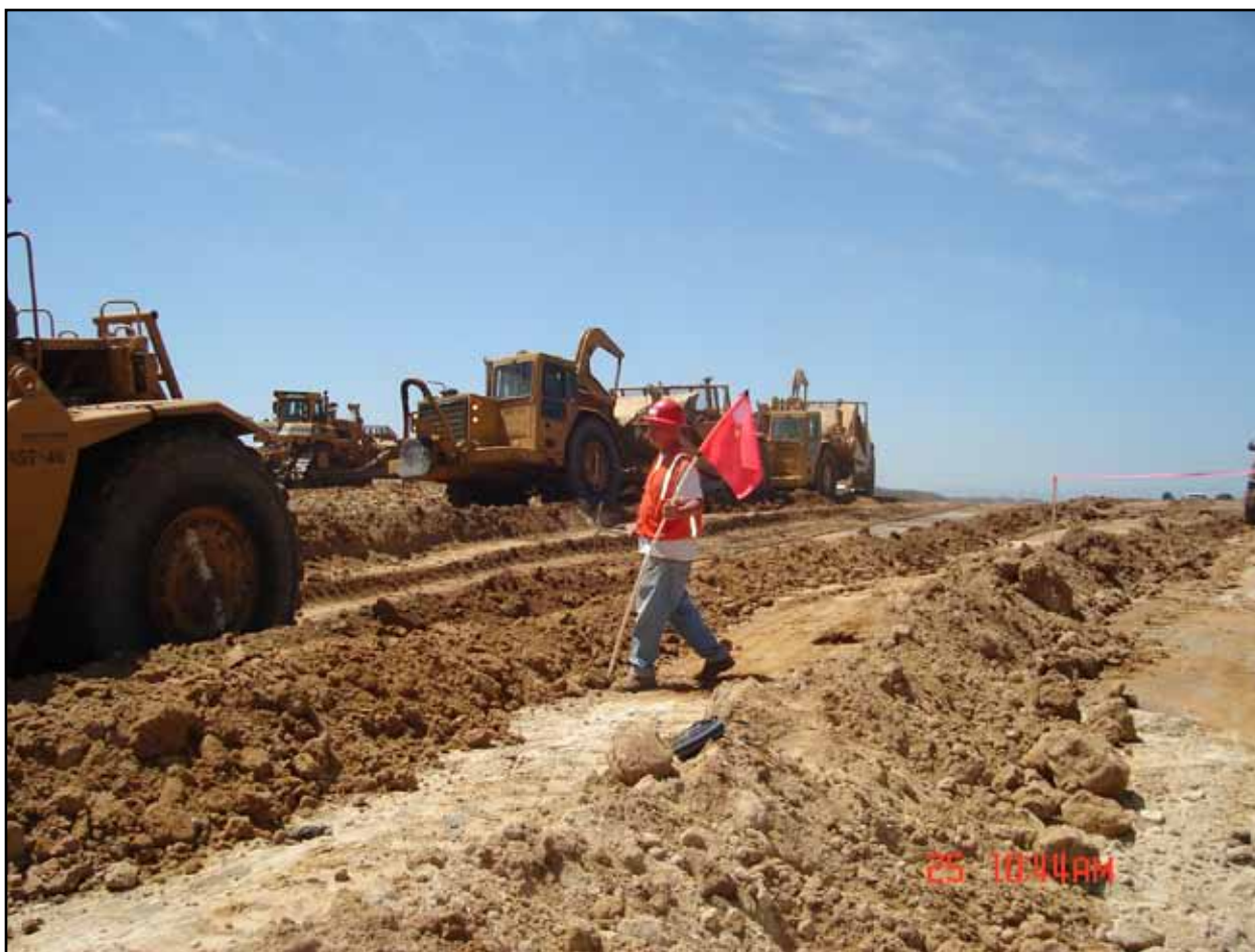
FIGURE 3. Field paleontologist Pat Sena monitoring mass grading activities in upper Pliocene strata of the San Diego Formation as exposed during construction of residential housing in coastal San Diego County. San Diego Natural History Museum, Department of PaleoServices photograph.
