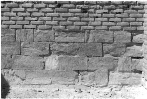
Stone and brick construction, Qasr al-Tuba, Jordan
