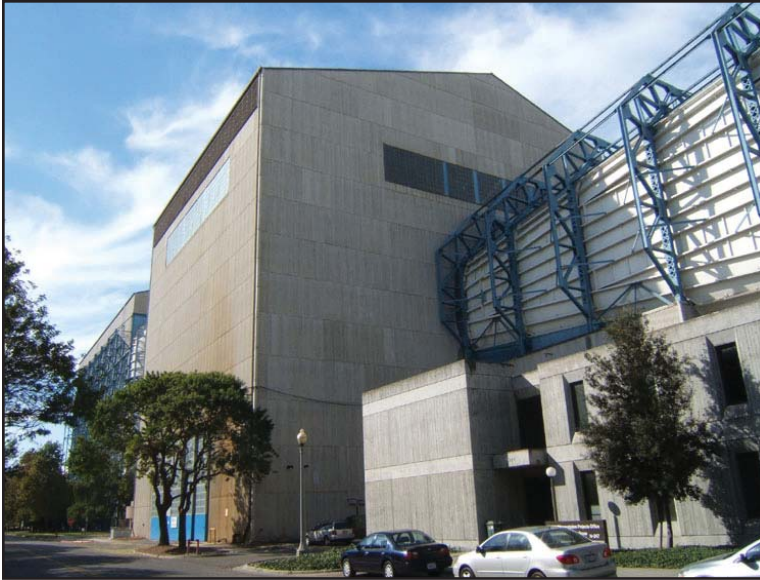
N-221, east facade (Source: Page & Turnbull)
