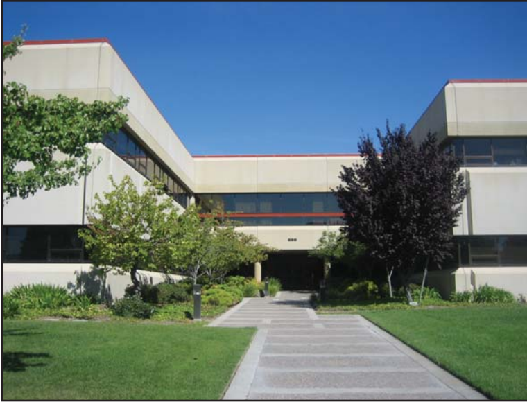
N-258, south facade, main entrance (Source: Page & Turnbull)
