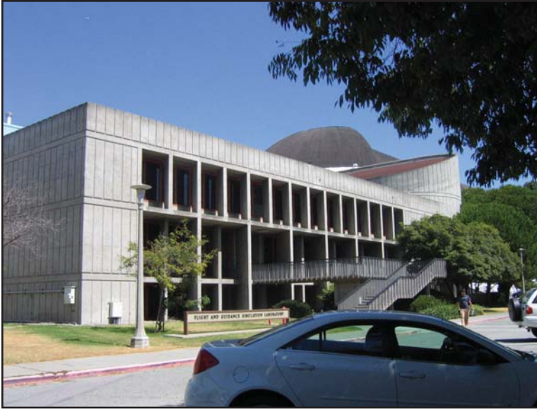
N-243, east facade (Source: Page & Turnbull)
