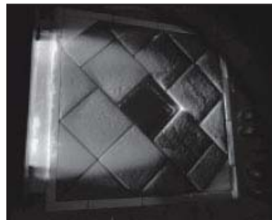
Figure 9. "Missing tile" heating test
