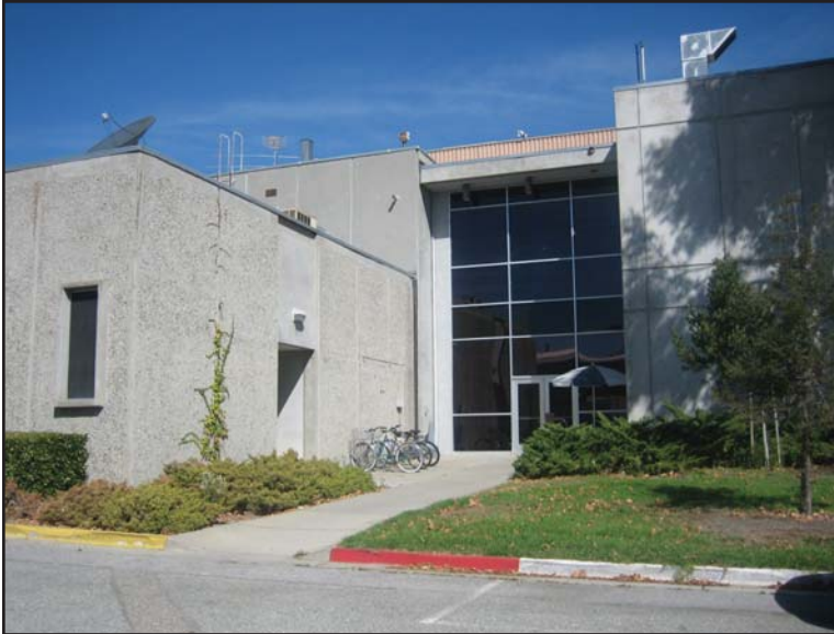
N-240A, main entrance (Source: Page & Turnbull)
