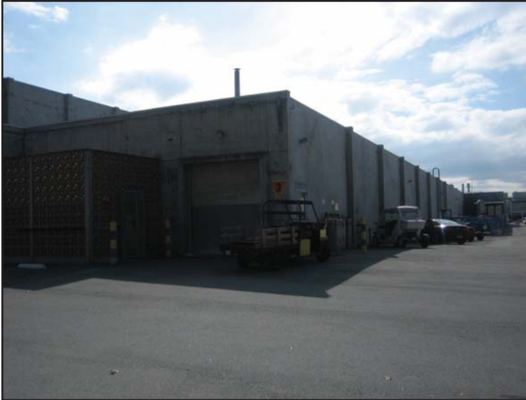
N-237, north and east facades, entrance to Hypervelocity Free Flight Facility (Source: Page & Turnbull)
