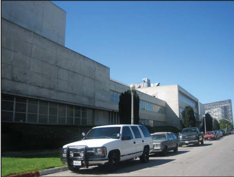
N-227, north facade (Source: Page & Turnbull)
