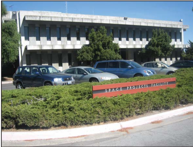
N-244, south facade, main entrance (Source: Page & Turnbull)
