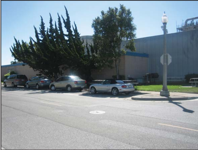
N-238, north facade (Source: Page & Turnbull)
