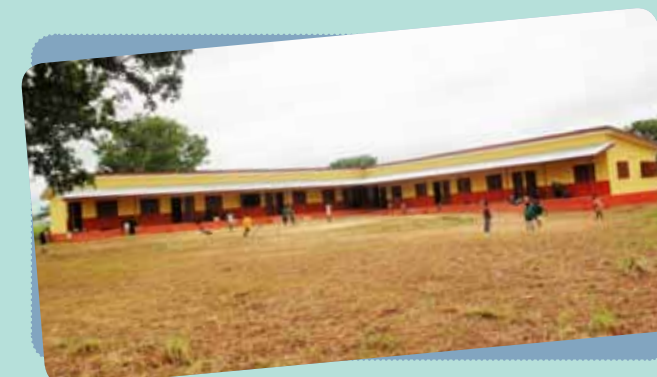
» Six Classroom Primary School Block
