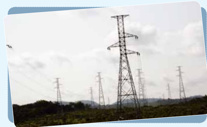
» Erection of Transmission Lines from the Bui Switchyard
