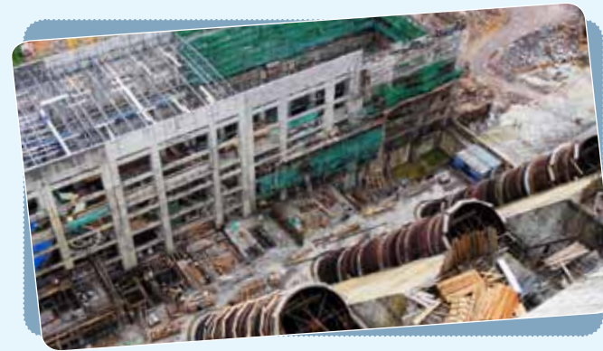
» Status of the powerhouse as of June 2012
