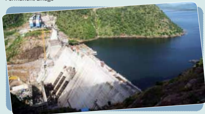
» Civil Work of Main Dam 95% Completed
