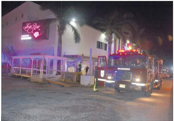
Late on Sunday the Fire Department had to respond to reports of a fire at Italian restaurant Sale & Pepe located in the Le Shore nightclub building (former Sunset Theatres) in Simpson Bay. An air-conditioning unit overheated and smoked out the restaurant, but owners managed to put out the fire before the Fire Department arrived. No injuries were reported during the incident, according to authorities.
