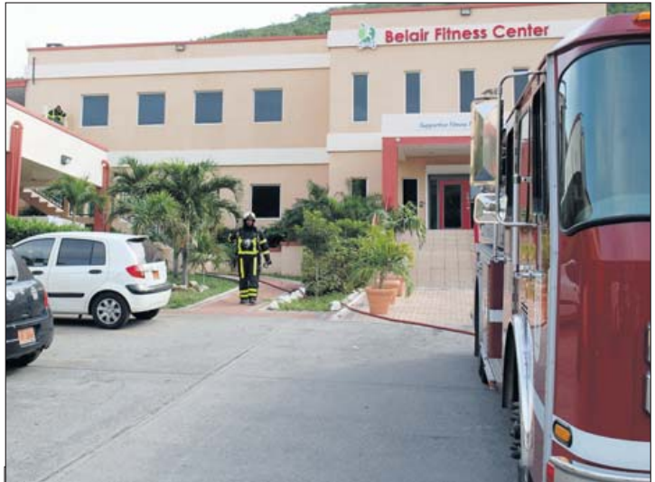
The Fire Department was called out when smoke started to come out of the Belair Fitness Centre on Monday morning close to midday. According to the fire-fighters, the smoke was a result of a mechanical failure coming from the pool area. The gym was not evacuated by the management because of the minor incident.
