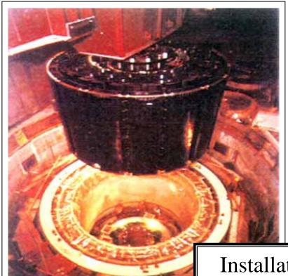
Installation of 266MVA ACG for 2units(Rotor)
