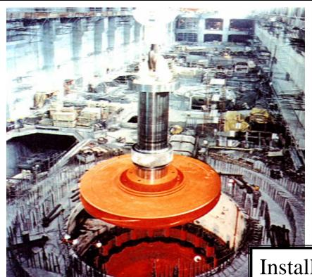
Installation of 260MW WT-G for 4units (Pump-Turbine)
