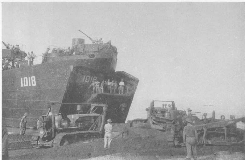
No. 3 Airfield Construction Squadron at the Mindoro landing on 15th December 1944. Men of the unit are using three bulldozers to build a ramp from the beach to the open bows of an LST.
