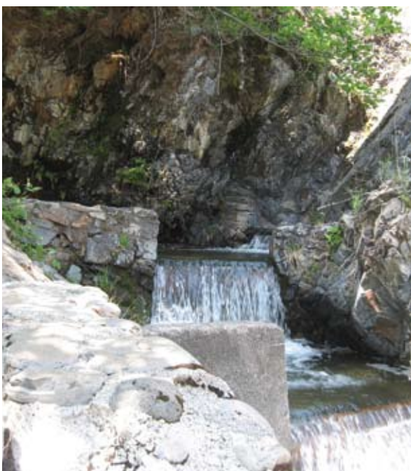
Fish ladder on Lower Deer Creek Falls
