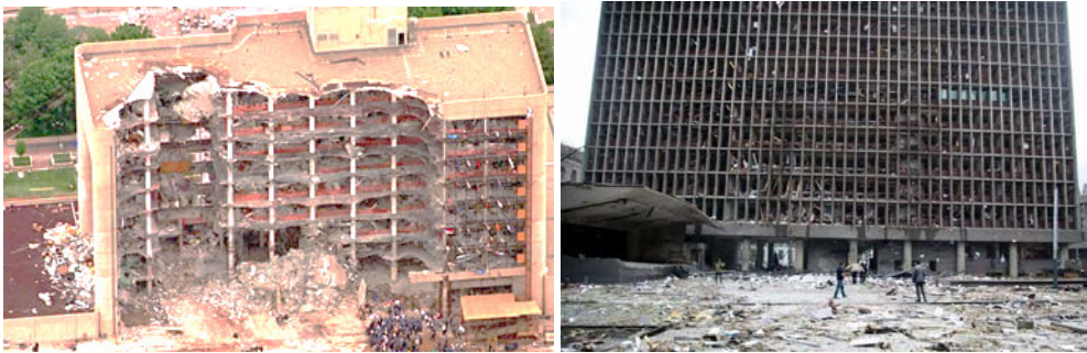
Figure 1a, 1b. 1a: Alfred P. Murrah Federal Building in Oklahoma City; 1b: Government buildings shattered in Oslo
